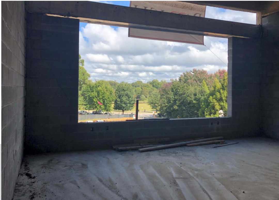
CMU Walls Installed on 3 rd Floor Classrooms Facing Piedmont Park
