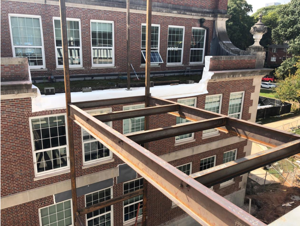
Steel Erection for New Addition Bridge Tie-In Progress
