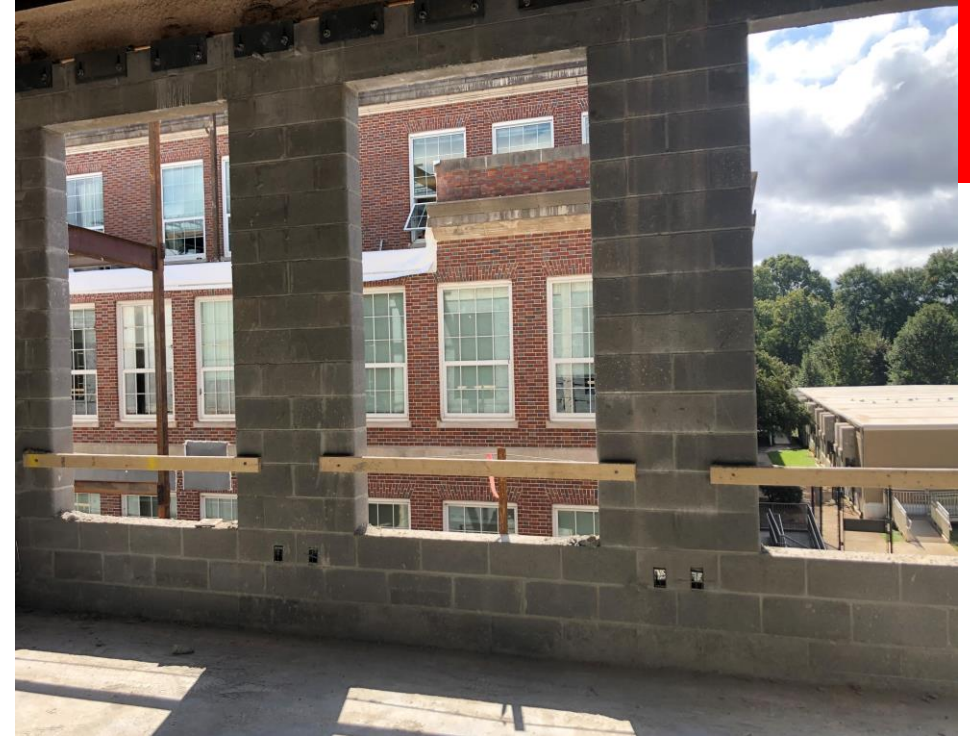
CMU Walls Installed on 3 rd Floor Classrooms Facing the Charles Allen Building
