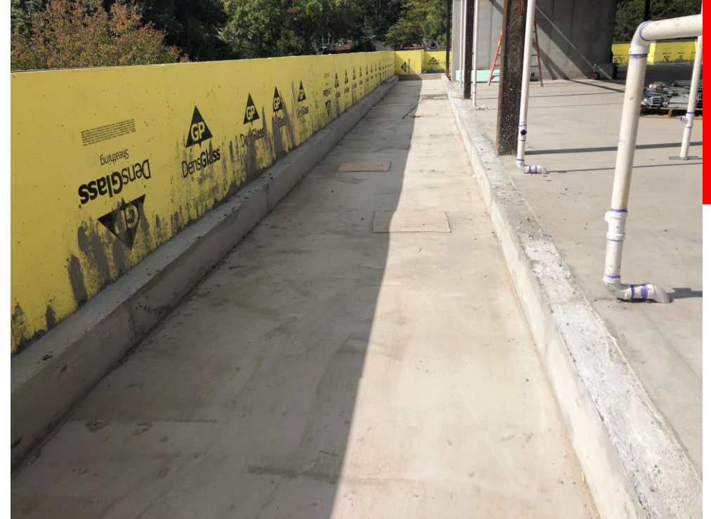
Concrete Curbs Poured at Fourth Floor Patio
